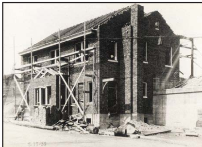
Construction of the Railroad Station photo submitted by Bob Sease
