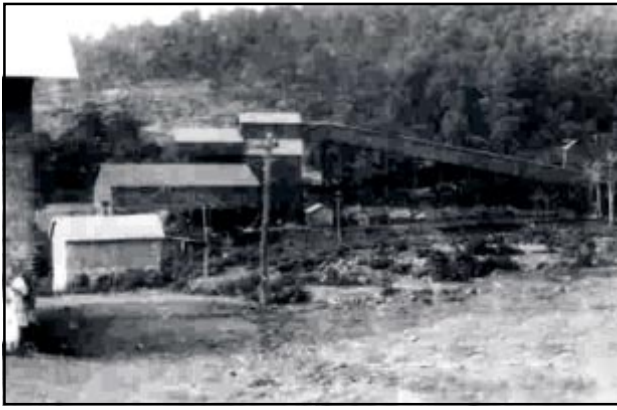
Puritan Mines - one of 58 mines in the Portage area
